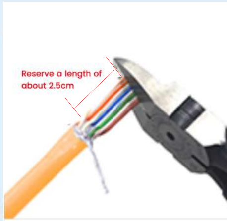
5. Cut the wires in oblique angle
