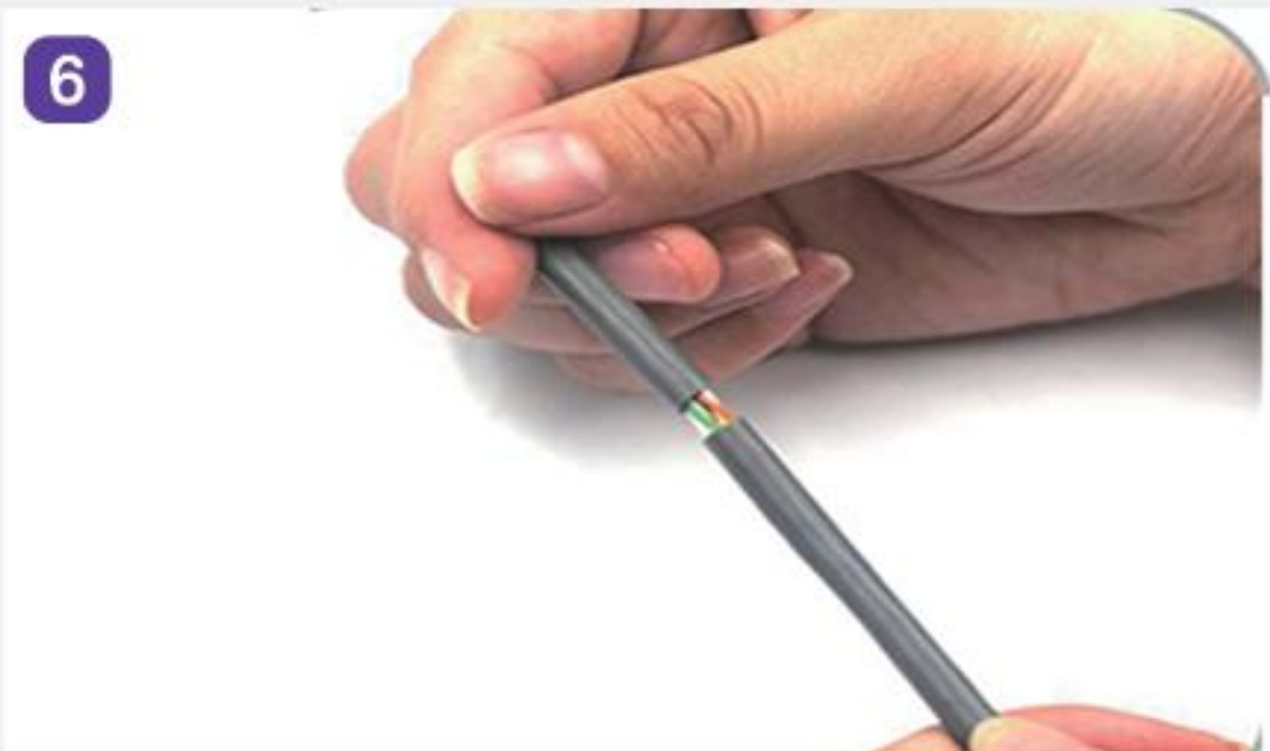
Pop the cable jacket.
